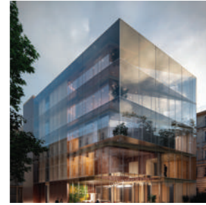
Public Buildings & HQ
